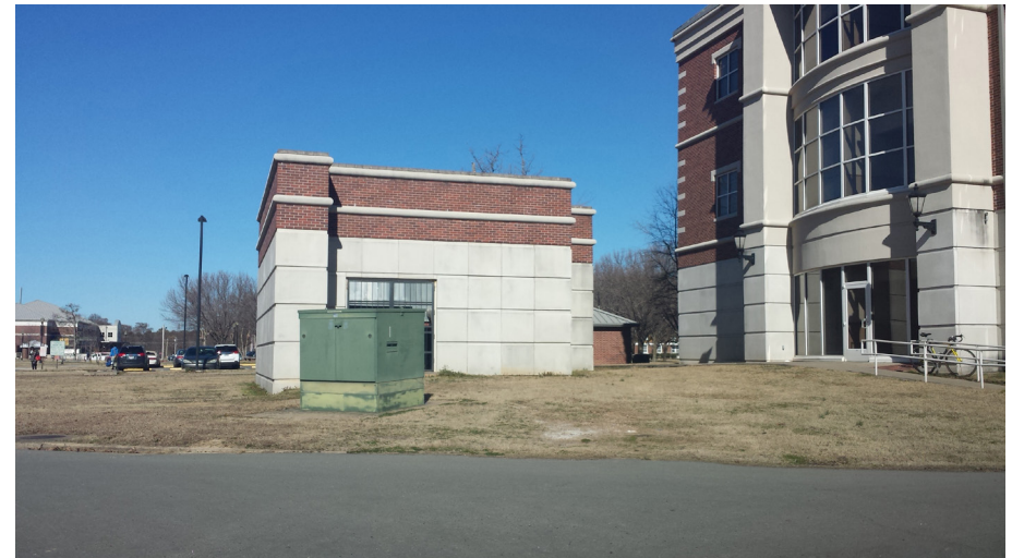
Figure 4.2-9, Mechanical Enclosure Building
