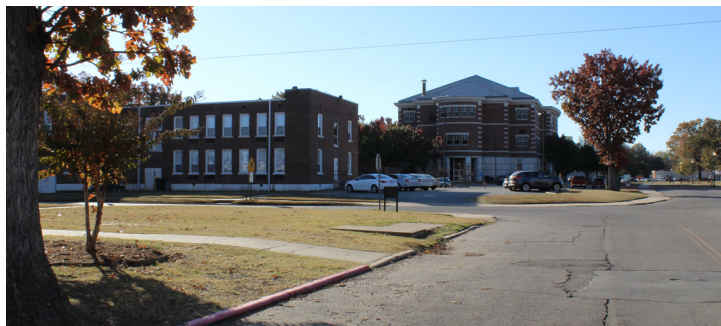
Figure 4.1-13, Existing Imagery of View of Pedestrian Mall Zone to Henderson_Young
