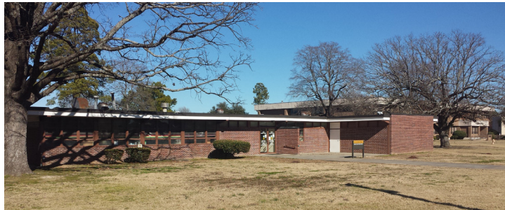
Figure 5.2-5, Demolition Planned for Browne Infirmary
