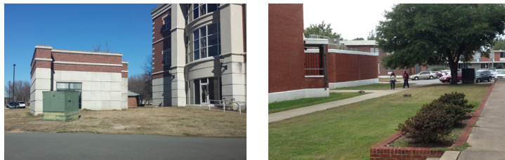
Figure 4.2-2, Examples of Existing Mechanical Enclosures around Campus
