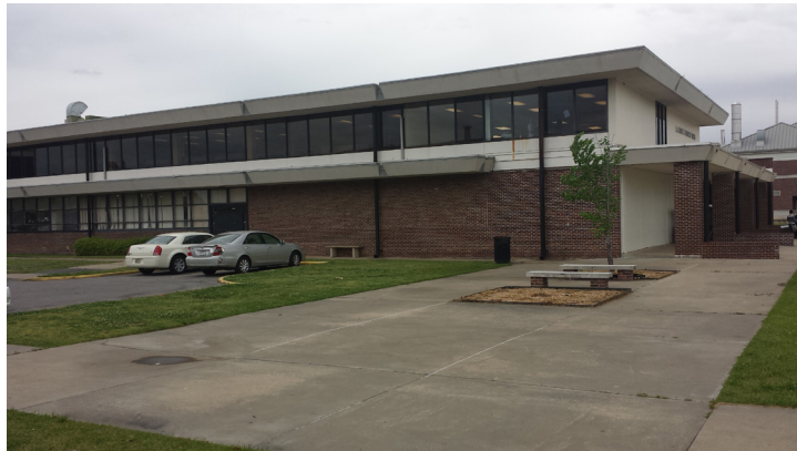
Figure 5.2-2, Renovation Planned for L.A. Davis Union
