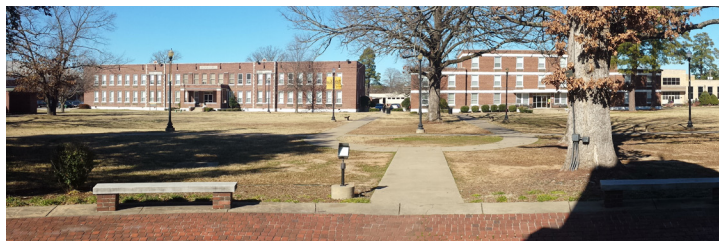
Figure 5.2-6, Demolition Planned for Lewis and Douglas Hall
